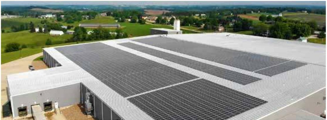
In 2021, we completed installation of a 1.792 MW solar array at our stone manufacturing facility, comprised of 4,480 solar panels. It is expected to reduce electrical power consumption by 60% and to prevent emission of 1,472 tons of CO<sub>2</sub> annually.
